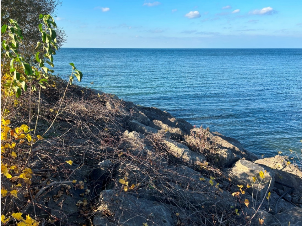
Photo 1: View of Revetment looking West
