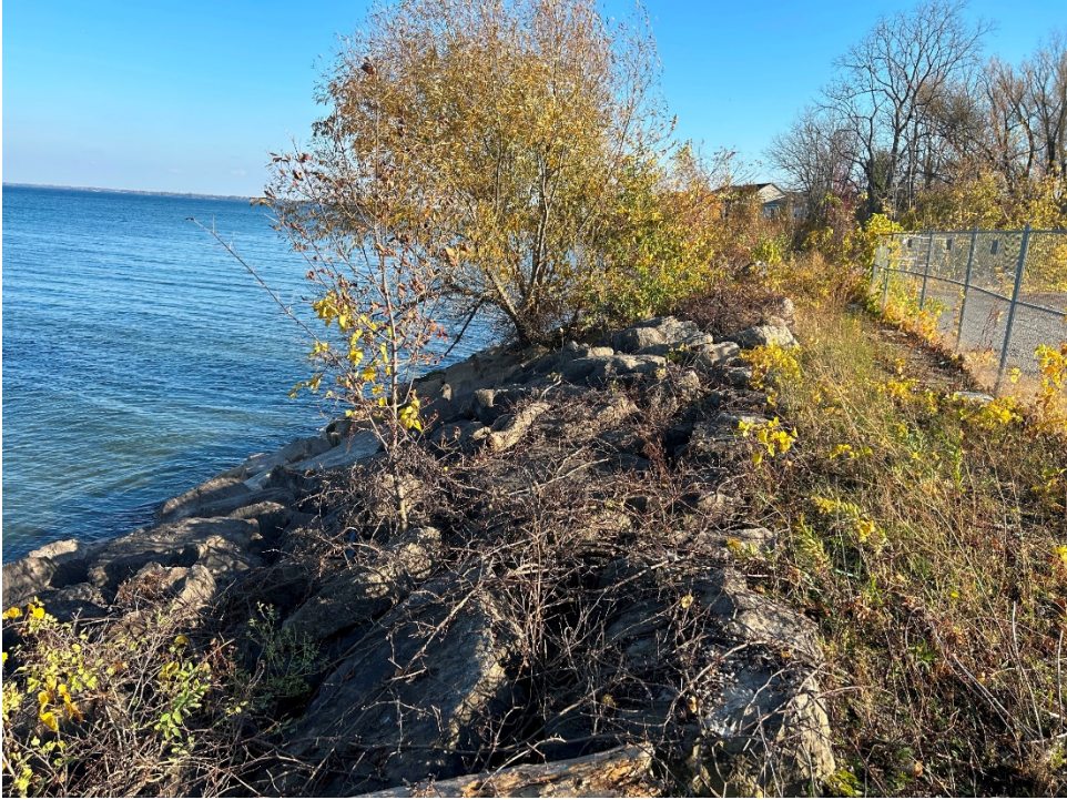
Photo 2: View of Revetment looking East
