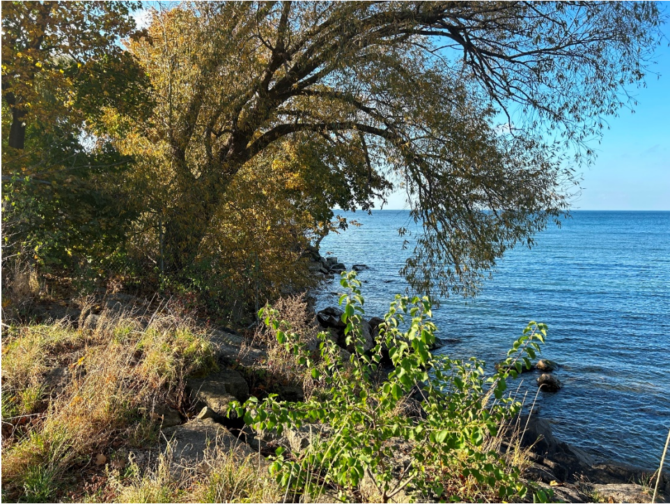
Photo 7: View of Shoreline Protection to the West
