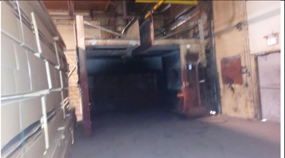
Photograph 8 Interior of Industrial building, paint booth.
