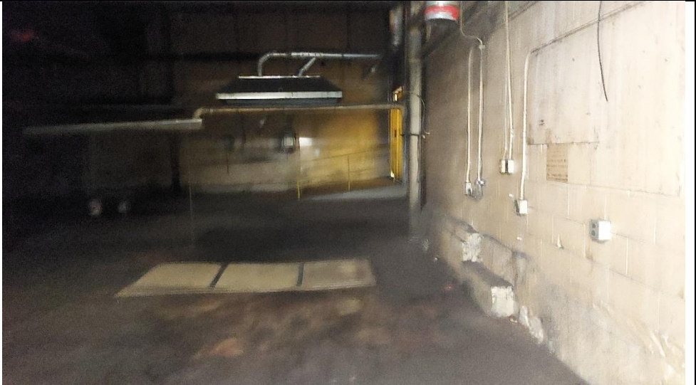
Photograph 7 Interior of Industrial building.
