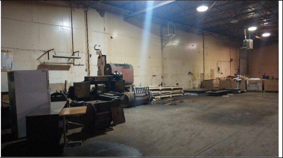
Photograph 10 Interior of Industrial building.
