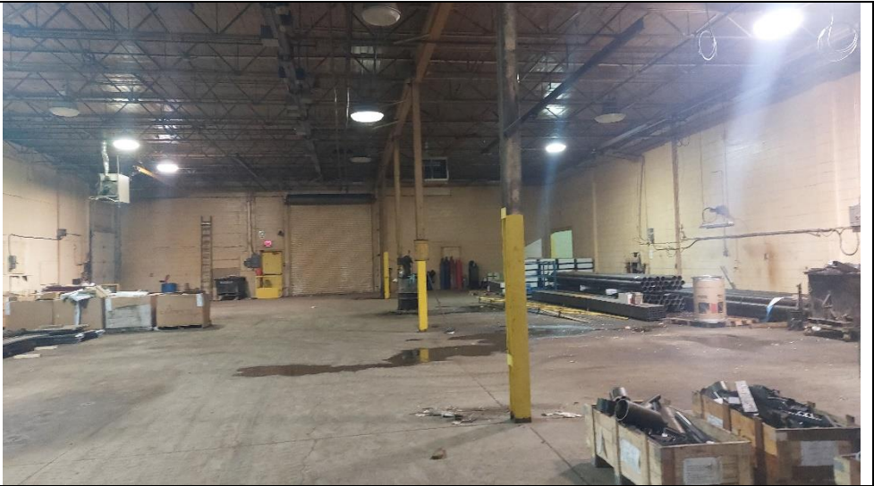
Photograph 9 Interior of Industrial building.
